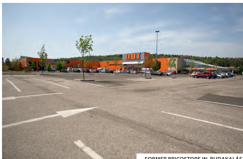
FORMER BRICOSTORE IN BUDAKALÁSZ
