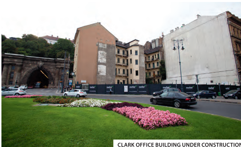
CLARK OFFICE BUILDING UNDER CONSTRUCTION
